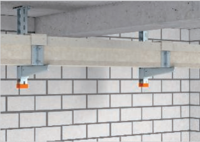
Suspended ceiling mounting as I duct.
