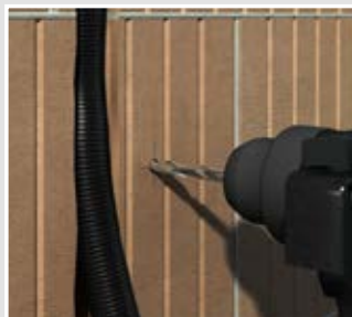
Cut Ø 8 mm drill hole at least 50 mm deep.
