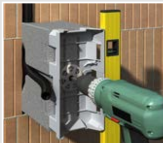
Hold the equipment carrier against the wall, align it, and fix it using the dowel.
