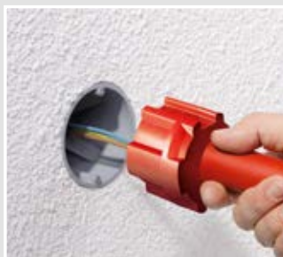
Use KAISER tool Styro55 for fast, easy fitting of the swivels.
