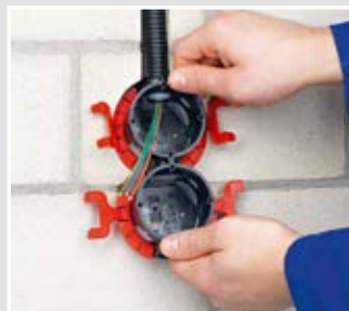
Push in box with Klemmfix® clipped on.
