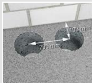
The ceiling penetration sealing systems can also be arranged as a group with a distance of 205 mm or 125 mm.
