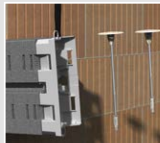
Remove the side lugs from the screw dowel. Note the different lengths!
