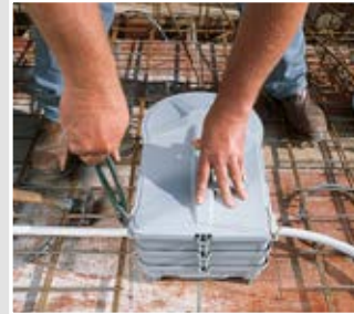
Also secure the housing to the reinforcement.
