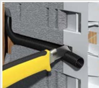
Press the conduit into the side guide and cut it to length.
