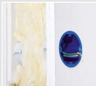
Use of an opposing sound insulation box.
